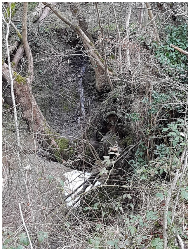
Seepage through made ground creating small waterfall
