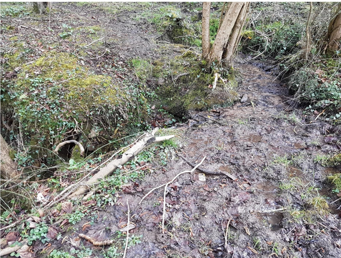
Saturated made ground/seepage
